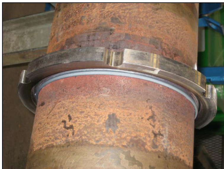
Figure 5. Visual examination of weld 2
