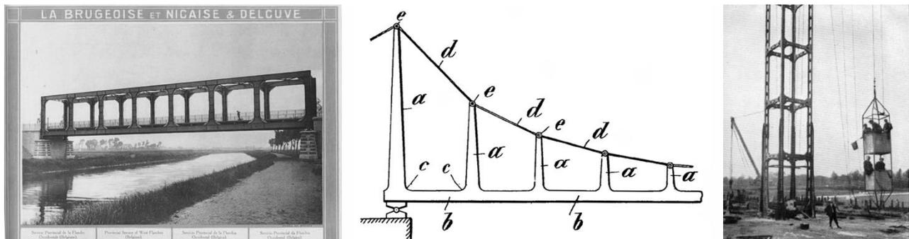
Figure 2. Vierendeel's first large bridge in Avelgem built in 1904 (contractor's catalogue); A concrete suspension bridge (Vierendeel [29]); A 287 m high radio pylon in Ruiselede (Jadot [4]).
