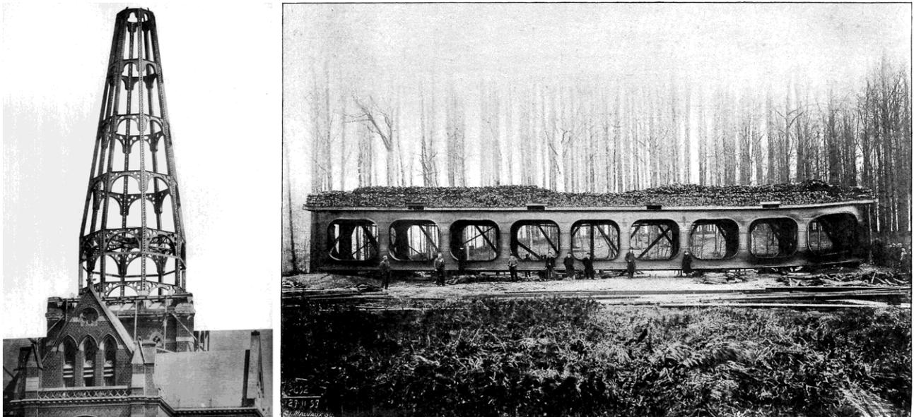
Figure 1. Framework of the crossing tower of the Dadizele church (Vierendeel [27], pl. 94) and Vierendeel's experiment of Tervuren in 1897 (Lambin, Christophe [6]).
