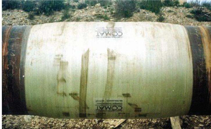
Figure 3: Composite crack arrester used in the Demopipe project
