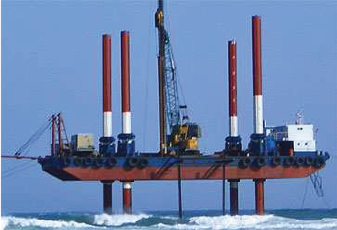
Figure 3: Jack-up barge supported by four tubular legs
